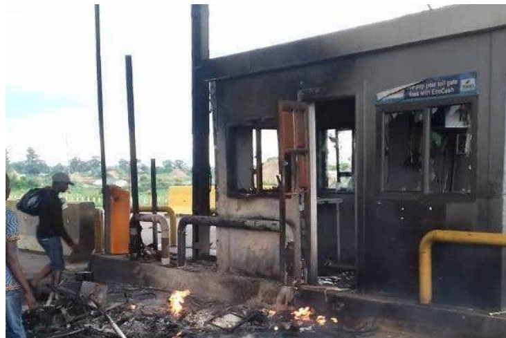
Figure 2: Masvingo tollgate damaged by protestors in January 2019 9 .
